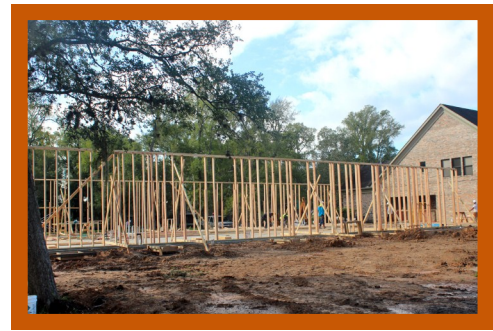
Framing of the First Floor Walls
